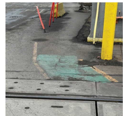
Pedestrian Crossing: Designated walkway painted on the pavement
